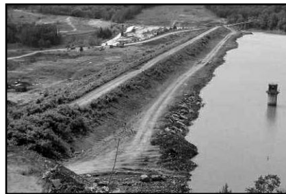
Buttress on upstream side of the Lake Fort Smith Dam.
